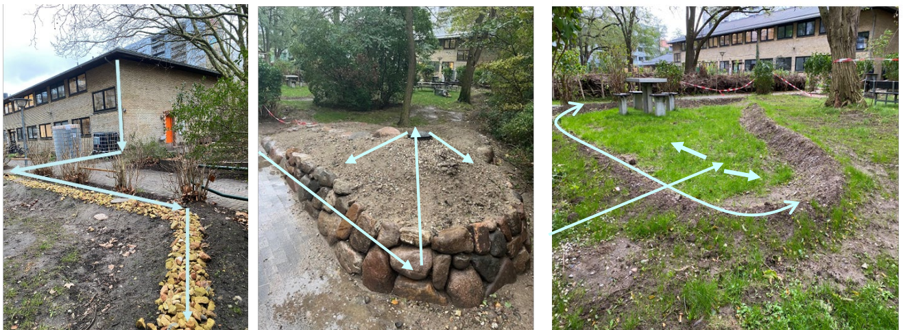
Figure 2: Left: Photo of the Rain Dike, receiving runoff from 45 m 2 of roof. Middle: Photo of the Rain Mound, receiving runoff from 65 m 2 of roof. Right: Raised Rainbed, receiving stormwater from 80 m 2 of roof. Flow marked with blue arrows.
